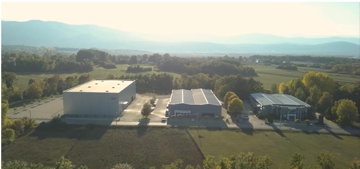
Lumen d.o.o. - headquarter, factory and central warehouse in Drinovci, Bosnia and Herzegovina
